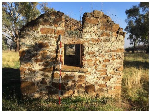
Plate 63. East wall with window and square shape missing at the top of the gable of outbuilding (West)
