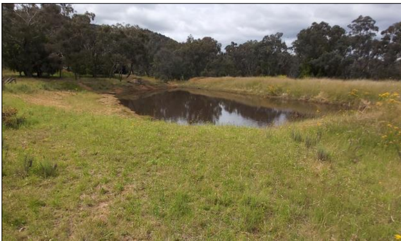
Drainage pond north of Oldfields Lane.
